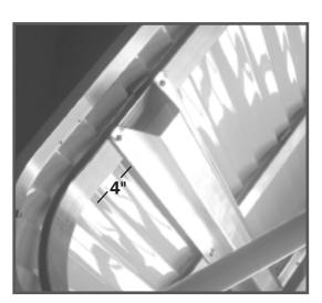
The hat section should be flush on each end of the outside rafters.
