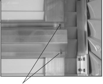
**3)** Drill holes using 1/8" drill bit. Two holes per rafter. One on each side of the "hat".
